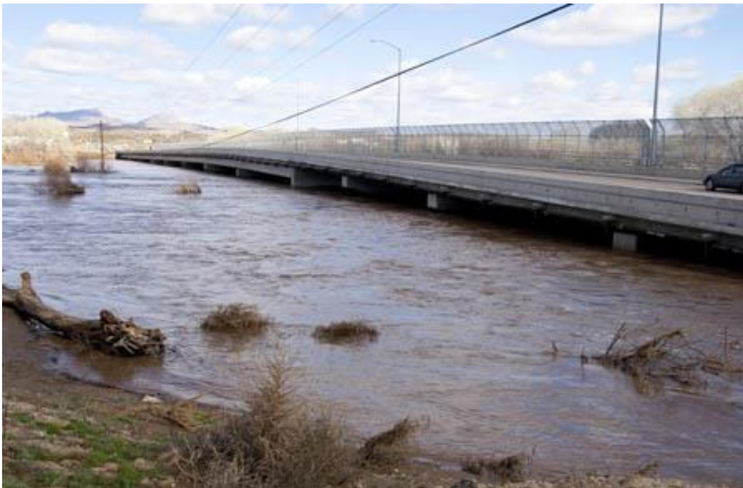
Figure 3.2: Downstream Side of Bridge [4]
