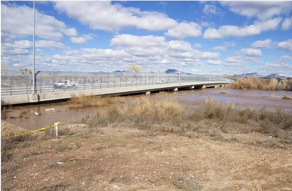
Figure 3.1: Upstream Side of Bridge (Fence) [4]
